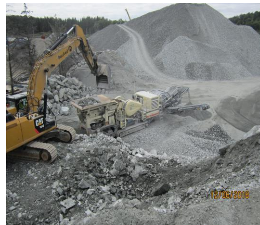
Mobilt knuseverk, Hordaland
