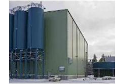
Boliden - Garpenberg, Sweden 130 m 3 /hr, 2005
